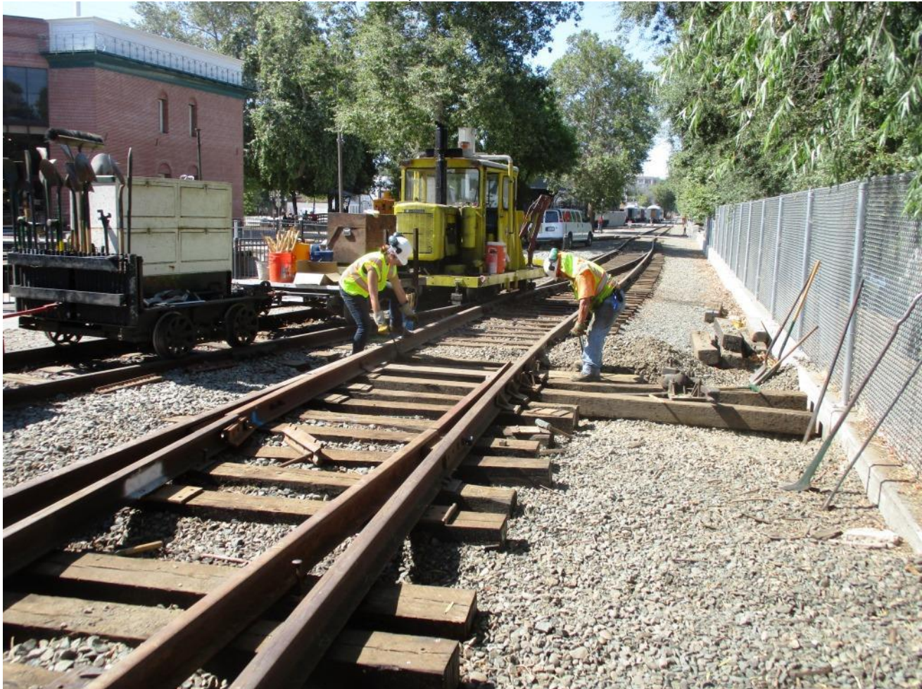
Samantha and Joe get the tie under the rails without mechanical assistance
