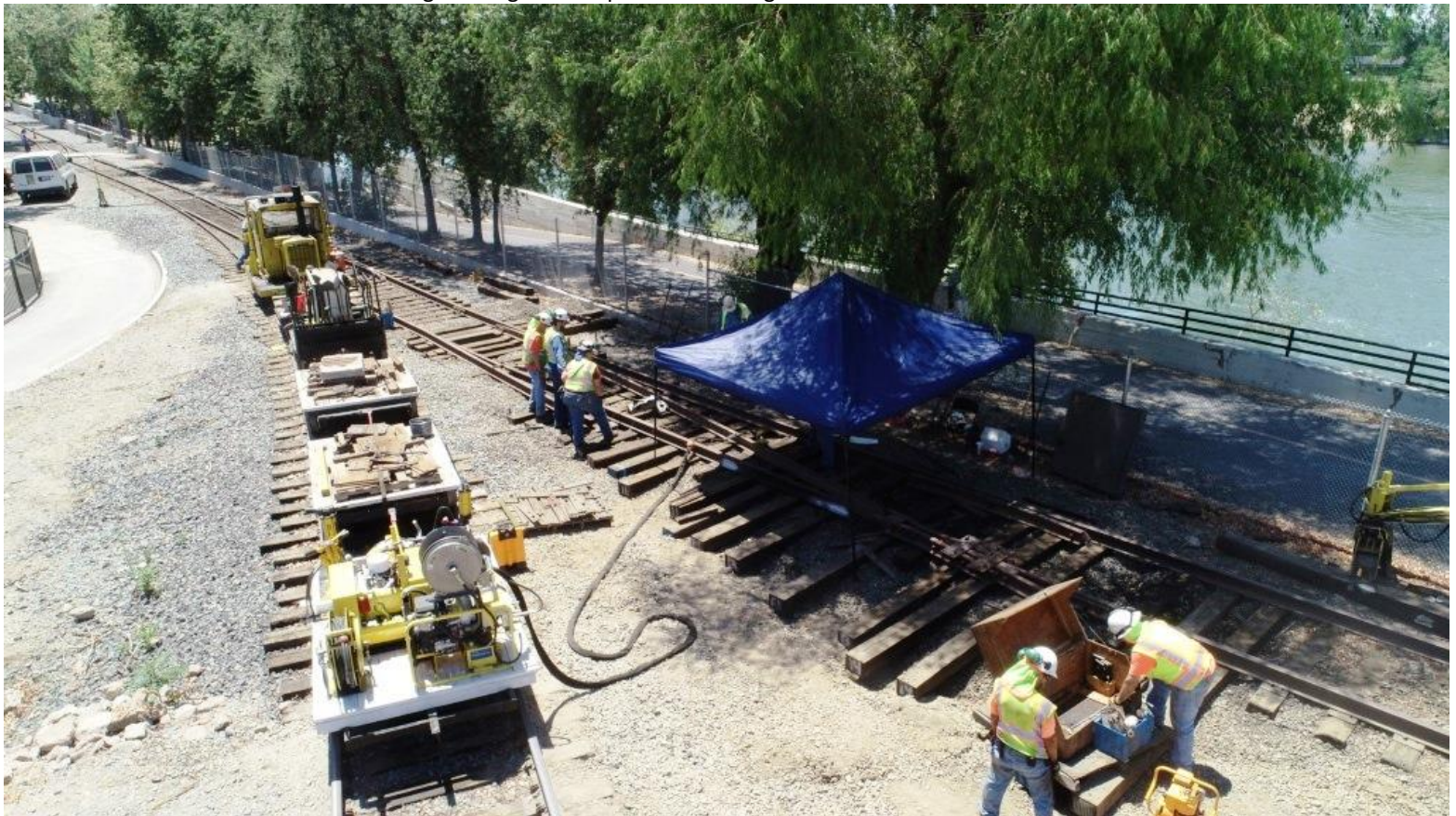
Bill, Weston, and Heather (center left) work on curving the closure-rail as Joe and Mike H. (lower right) deploy the rail-drill
