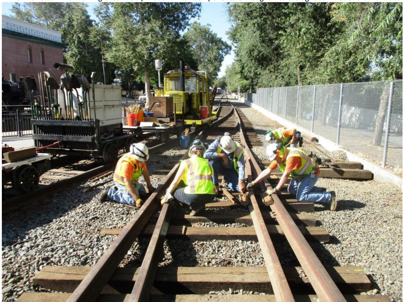
Mike H., Samantha, Alan, Bill, and Joe remove the heel-blocks installed last week to replace them with the modified blocks
