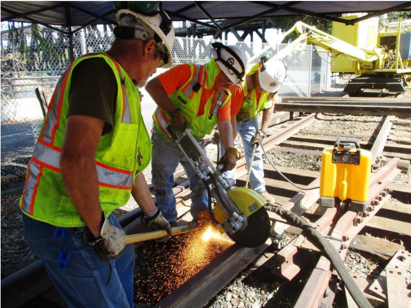
Ed shields sparks as Mike H. cuts the closure-rail to fit with the frog and Bill stands ready with the water pump
