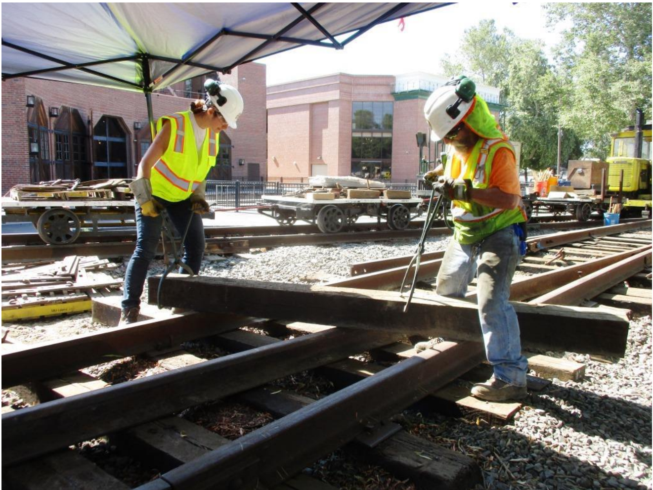
Samantha and Joe prove that they don't need a machine to move and insert a tie
