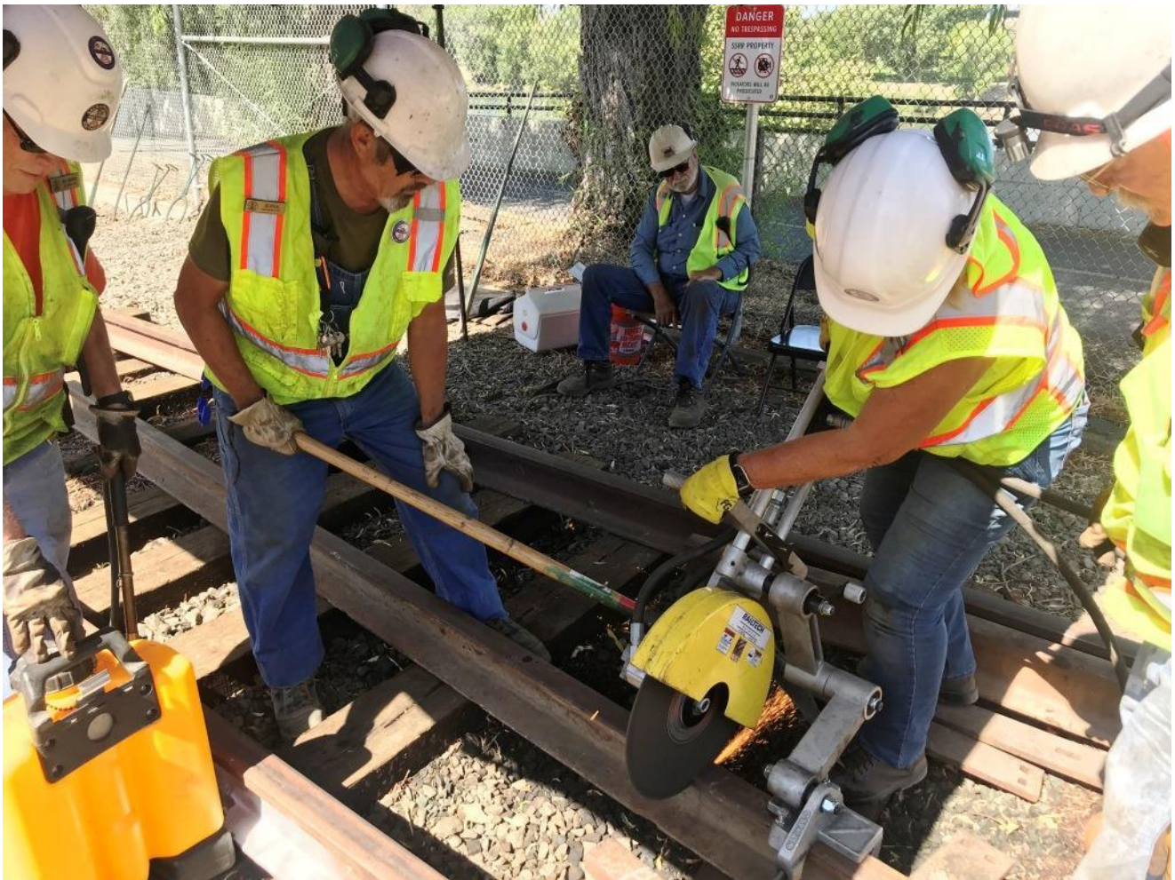
Next, Bev takes over on the rail-saw and slices away at the closure-rail
