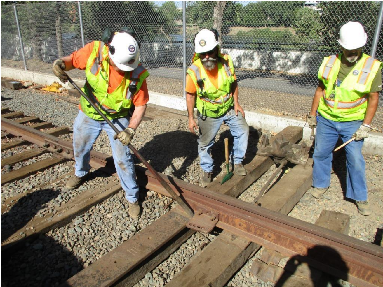
Bill, Joe, and Ed work on moving the head-block to center the switch-points over the gauge-plate
