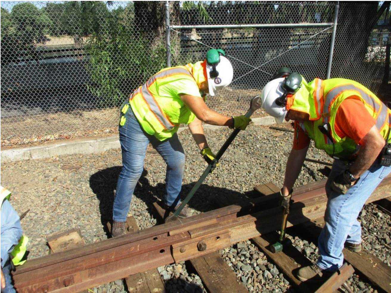
Bev and Bill and connect the closure-rail to the heel-block and tighten the bolts
