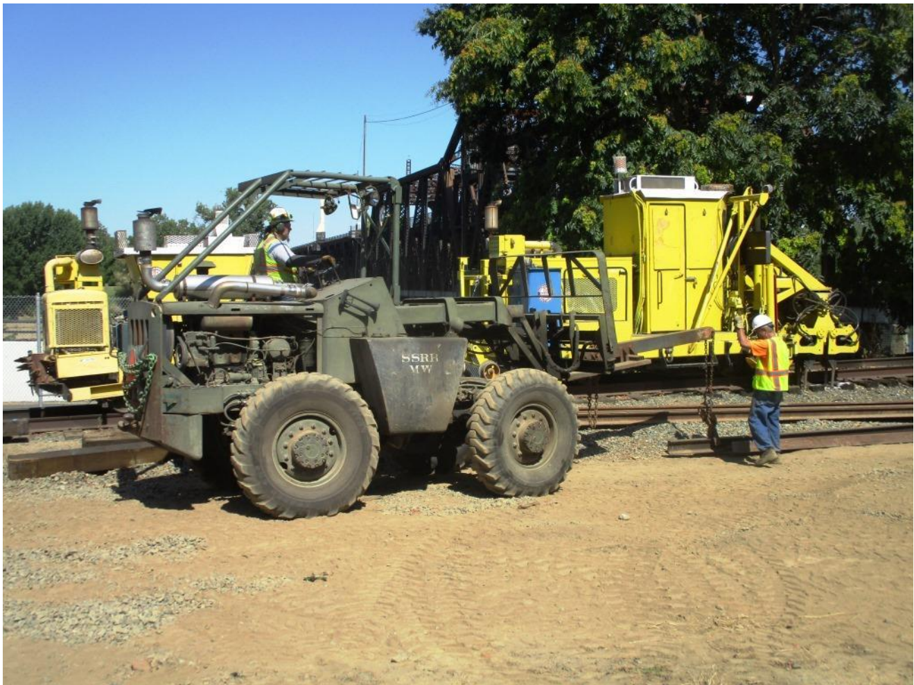
John directs Mike F. on Big Green as rail is moved in preparation for building the storage track
