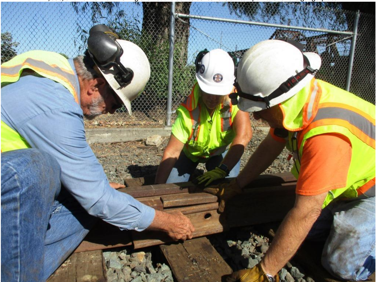
Alan, Bev, and Mike H. reassemble the heel-block on the west rail
