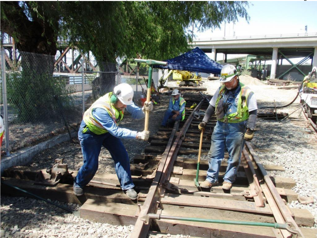
Despite the availability of modern technology, Weston and Mike F. interpret old-fashioned track-gang railroading by driving spikes by hand
