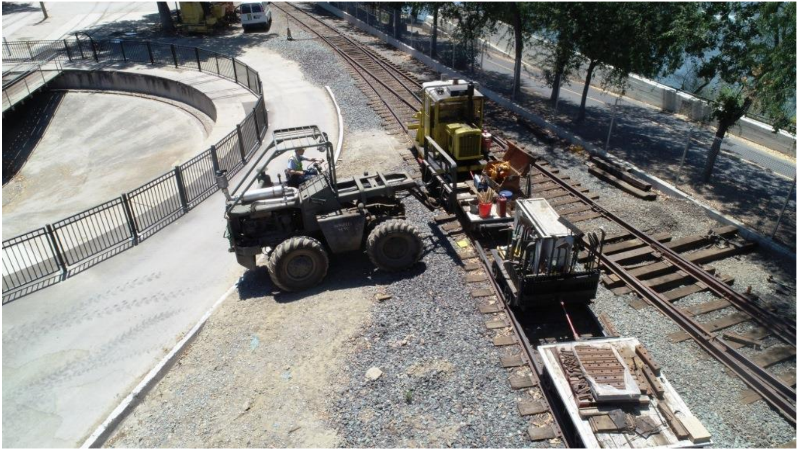
Big Green grabs the pallet containing the rail-drill off the flat-car
