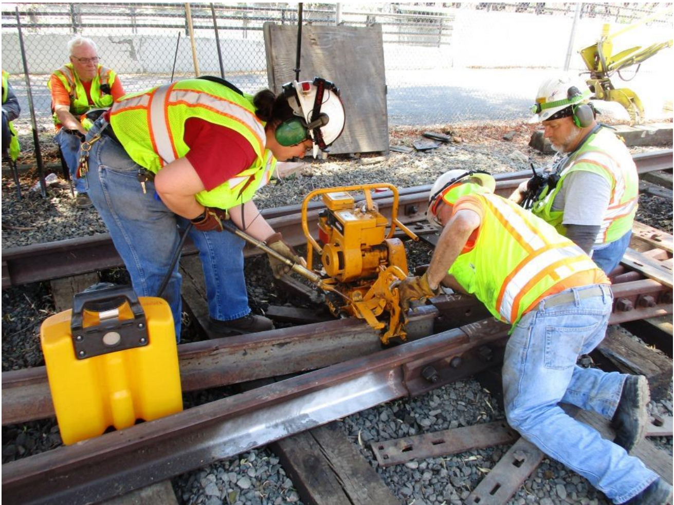
With the closure-rail sufficiently curved, Heather, Mike H., and Mike F. deploy the rail-drill to drill the bolt holes for connecting it to the frog
