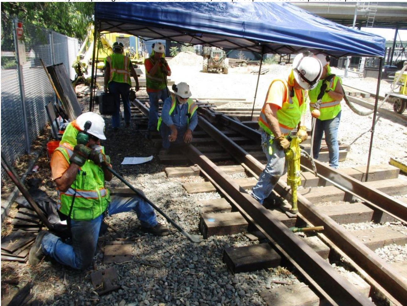
With the curve progressing, Joe nips the tie as Mike H. drives a spike with the hydraulic spike driver
