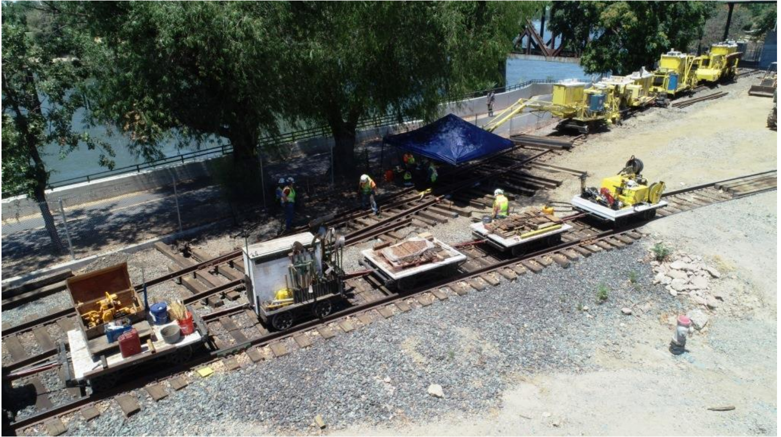
Ed uses his whirly-bird drone to capture some overhead shots of MOW Team's work-site
