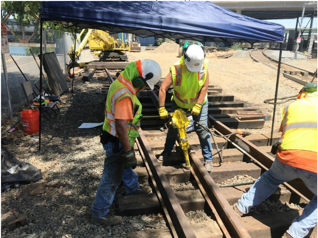
Bev drives spikes with the hydraulic spike-driver to hold the newly formed curve in the closure-rail
