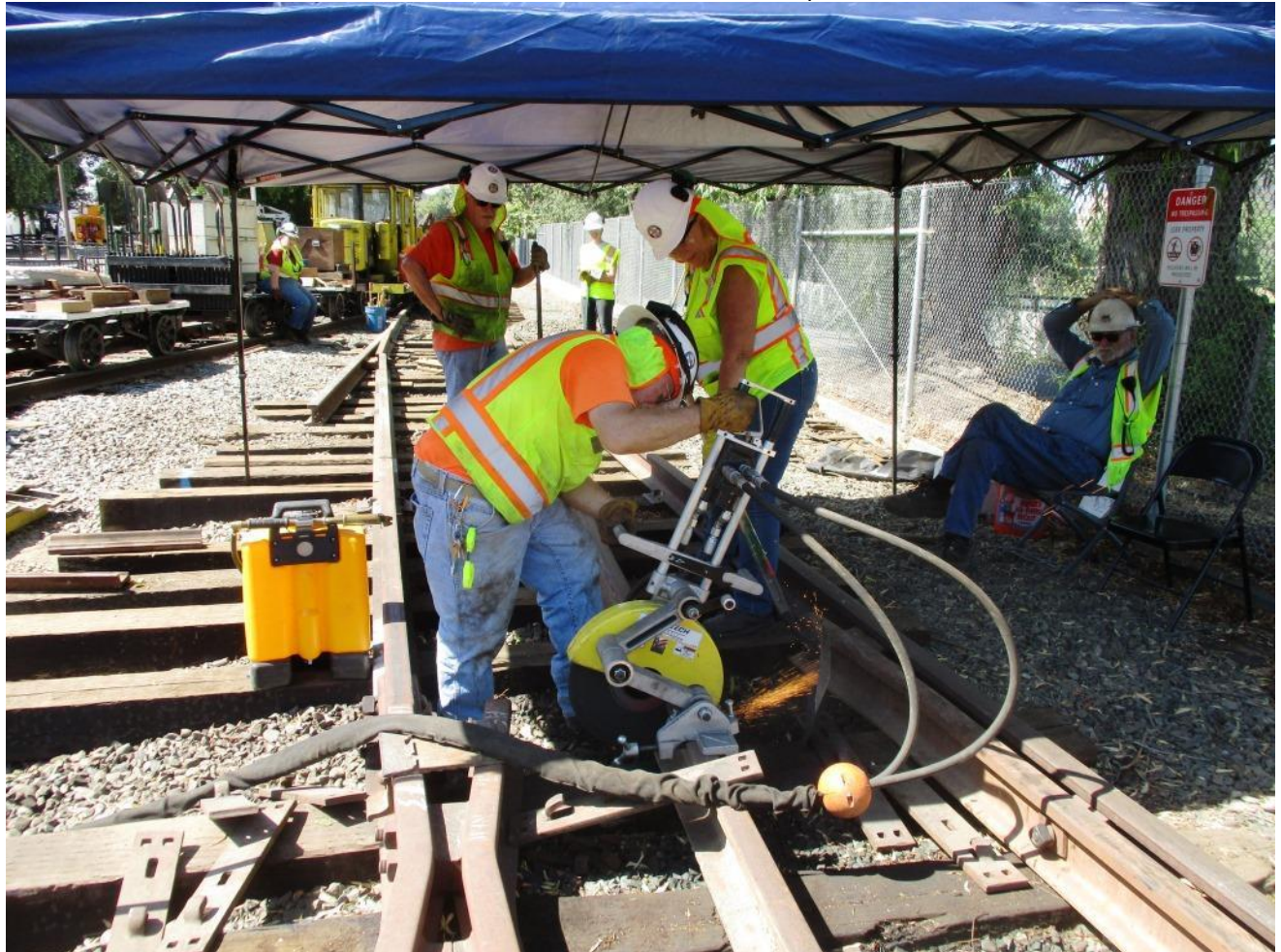
Bev shields sparks with the shovel as Mike H. makes the final cut
