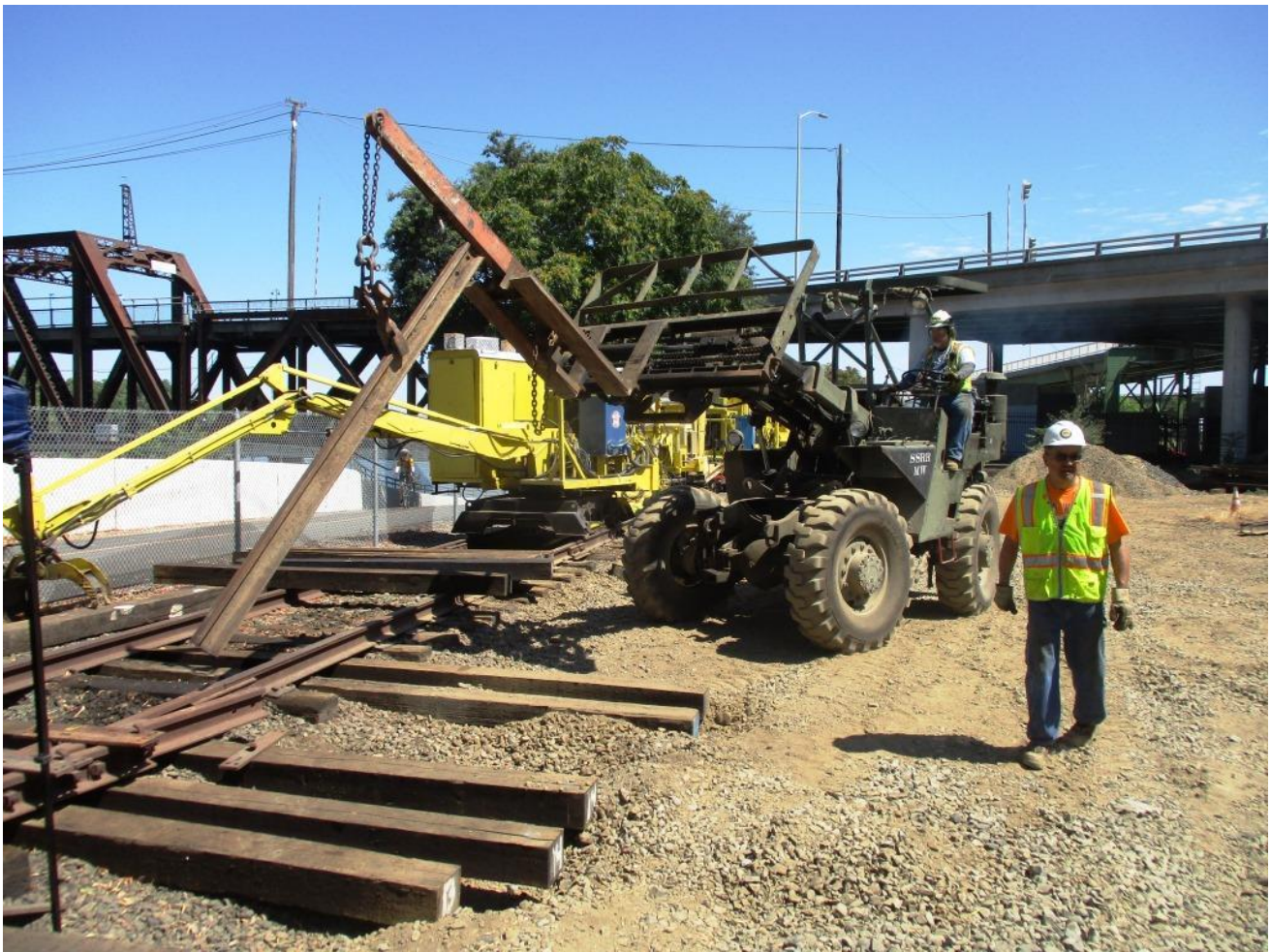
After the closure-rail is cut through, Mike F. on Big Green and John remove the superfluous section of rail
