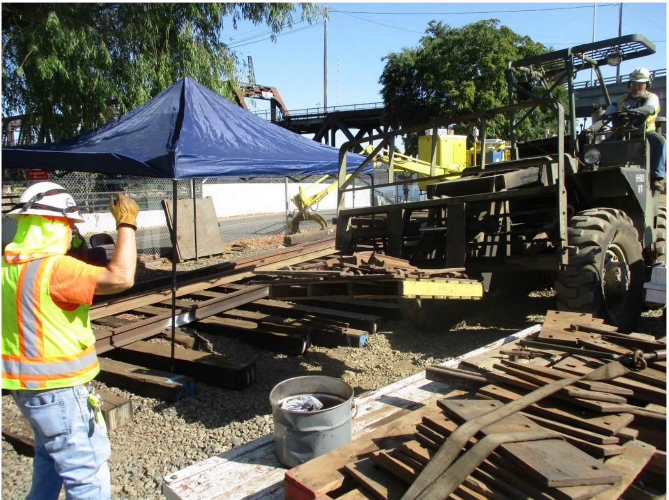
Mike H. directs Mike F. on Big Green as a pallet of switch components is brought into the tight confines of the work-site
